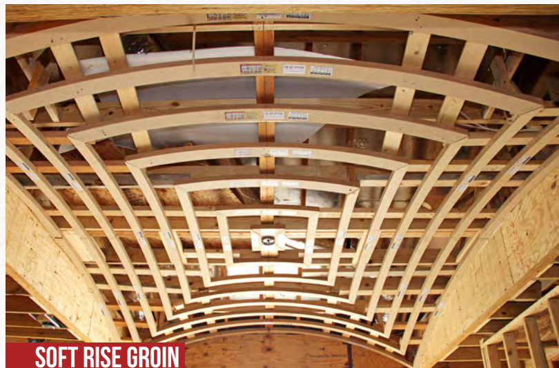
GROIN VAULT WITH BARREL EXTENSIONS
